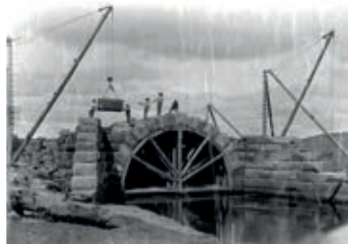
Photographs of stonemasons at work, France, circa early 1900s.
