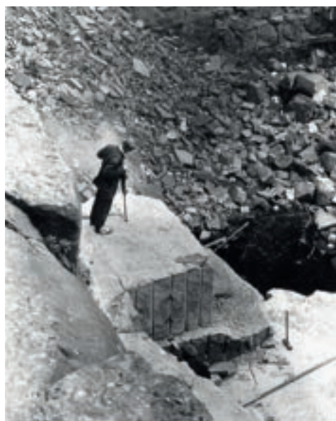
Top of page: Quarry blasting for cement production. Above: Traditional technique of drilling to split stone, circa early 20th Century.
